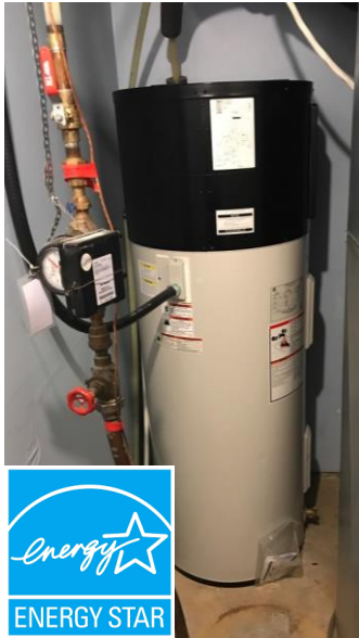
Heat Pump Water Heater
